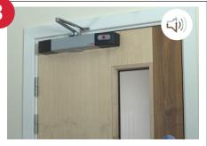
The Agrippa door closer recognises the fire alarm and automatically releases the door, protecting the building.
