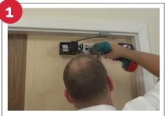
The Agrippa door closer is battery powered and wirefree. The device is installed at the top of the door.
