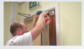
Align the keeper plate with the magnet face.
