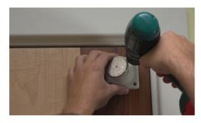
Check the rubber ring is fitted before screwing the keeper plate to the door.
