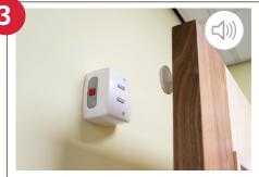
The Agrippa door holder recognises the fire alarm and automatically releases the door, protecting the building.
