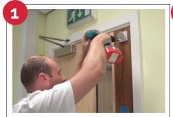
The Agrippa door holder is battery powered and wire-free. The device is installed at the top of the door and is pre-progammed to work.
