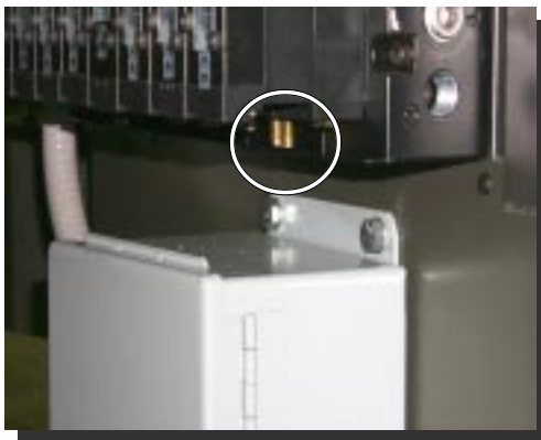
figure 17-3. Exhaust Restrictors
