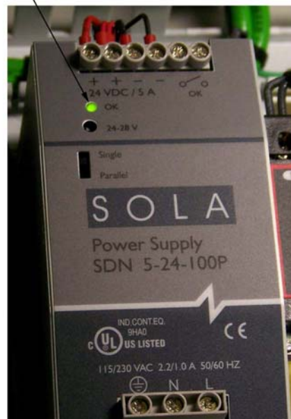
Figure 5-19 Power Supply Indicators
