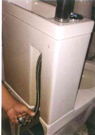
Step 4: Connect hot & cold water hose to the tap and connect the other end to outlet of the cistern.
