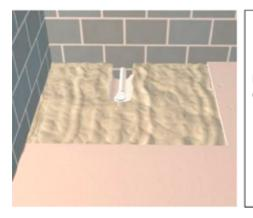
Lay a weak sand cement mix in the excavated area.
