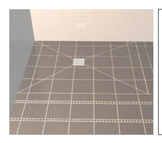
When the floor has been tiled and grouted, remove dust cover from the trap and refit the dip tube. Finally fit the grating into position.
