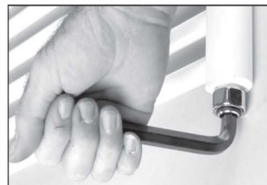
3. Tighten using an appropriate tool
