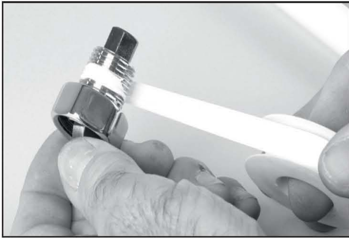
1. Wrap PTFE tape clockwise around the tail thread
