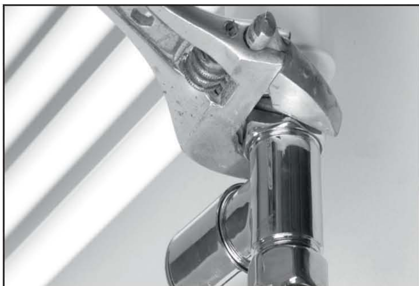
5. Fully tighten the valve using an appropriate tool
