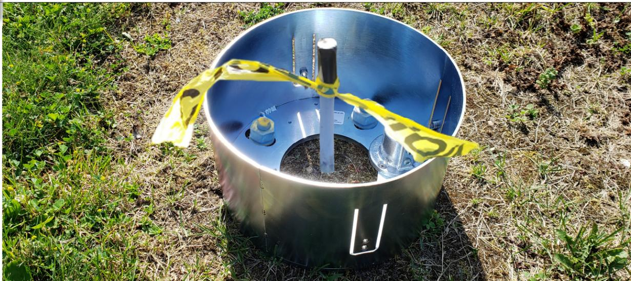
After the concrete has set, remove the bolt positioner board. Leave the lower nuts and washers in place for anchor base installation. Place the anchor base over the nuts. Level the anchor base, then fasten with another set of nuts and washers. Pull the data and power cables through the conduit.
