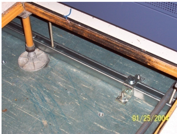
Subfloor bracing.
