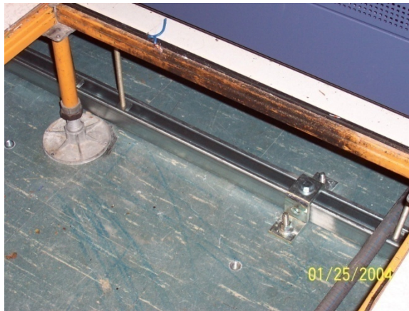
Fig. 2.2.1 Subfloor bracing
