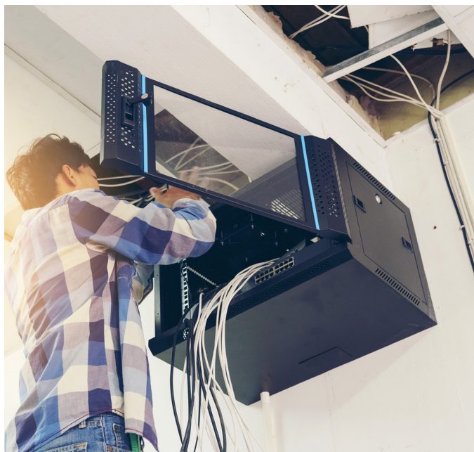
FIGURE 4: Installing cables in a zone enclosure.
