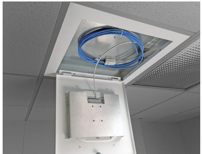
FIGURE 7: Example of a 2 x 2 ceiling mount opened, displaying properly stowed cabling and components for quick and easy authorized access without opening up the ceiling space. The quick-release interchangeable door provides a low-cost method of upgrading to future WAPs.
