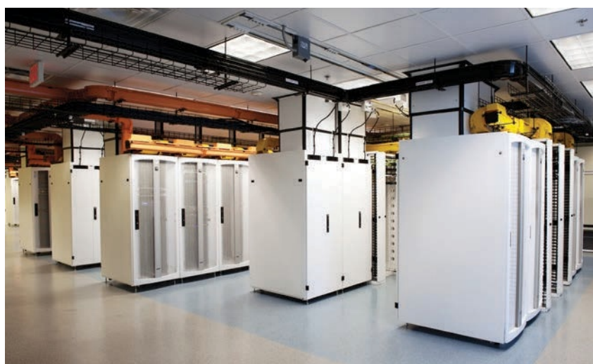
FIGURE 2: Hospital data centers rate an I_p of 1.5 because they cannot be offline following a seismic event.
