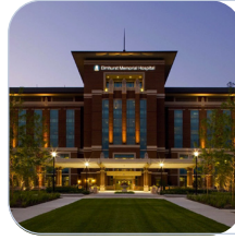
Elmhurst Hospital Elmhurst, IL
