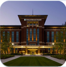
Elmhurst Hospital Elmhurst, IL
