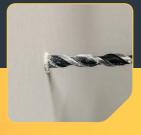
Drill a 13mm hole in the substrate. 50mm cavity clearance required behind substrate.
