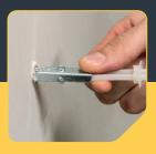
Ensuring the thumb tab faces upwards, insert the metal toggle through the hole, so it pivots down behind the substrate.
