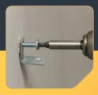
Insert a M6 screw through the fixture and into the threaded part of Zip-Fix and tighten until secure.
